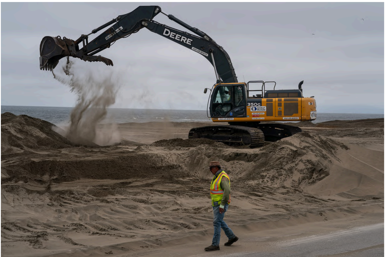
San Francisco Public Works personnel doing a sand-relocation project in 2023.
