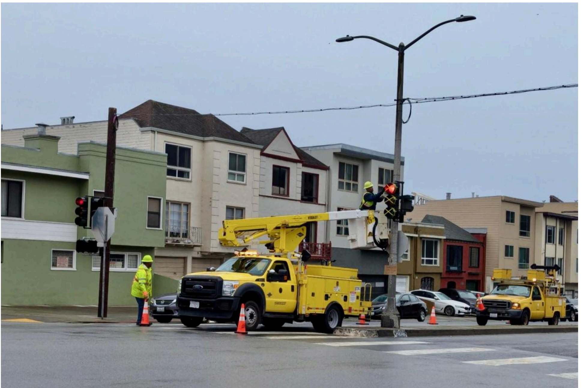
Our Signal Shop team activating the signal at 41st Avenue and Lincoln Way.
